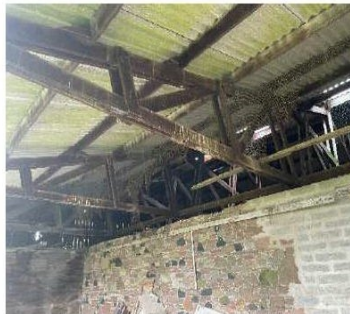
Figure 8.0 - View of timber roof trusses and roof sheeting
