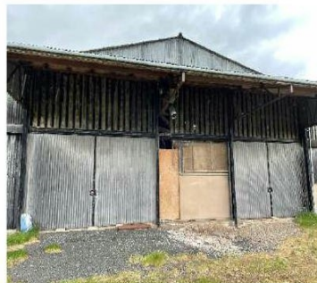
Figures 12.0 and 13.0 - Sliding doors with ventilation grille over
