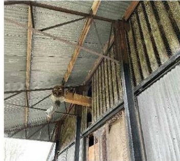
Figure 14.0 - Canopy Structure to East Elevation
