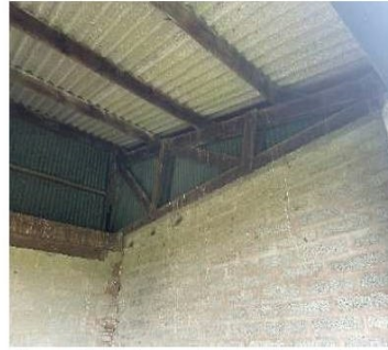
Figure 3.0 - Internal view of west elevation
