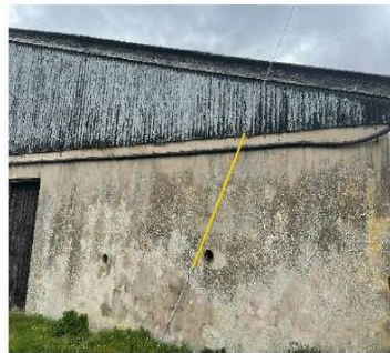
Figure 4.0 - View indicating small cores on southern elevation
